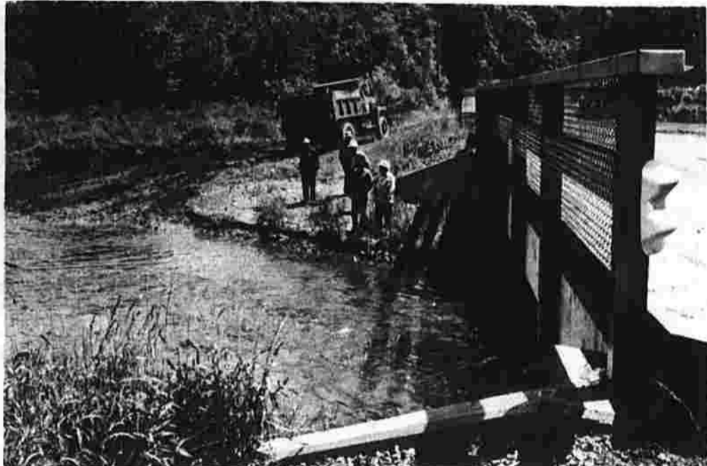
Silt dredged from under bridge
